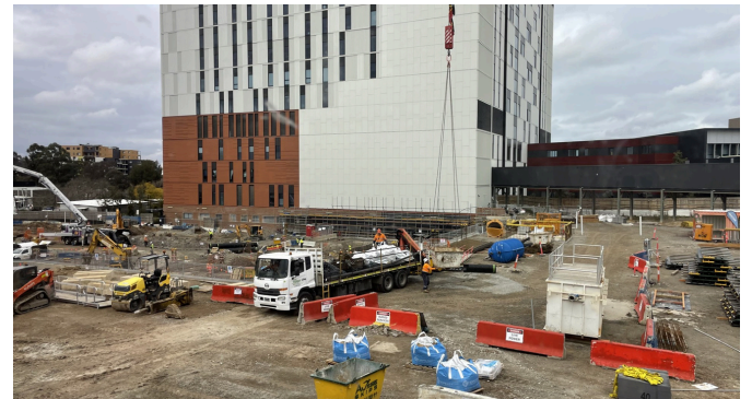
(Above) Works at the site of the new Stage 2 building
