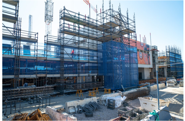
Outer edge of tower construction site
