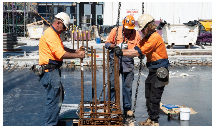
Workers on tower construction site
